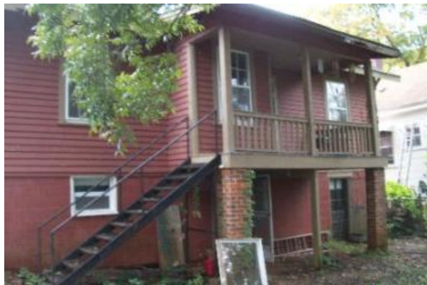
View of the rear porch with the metal stairs
