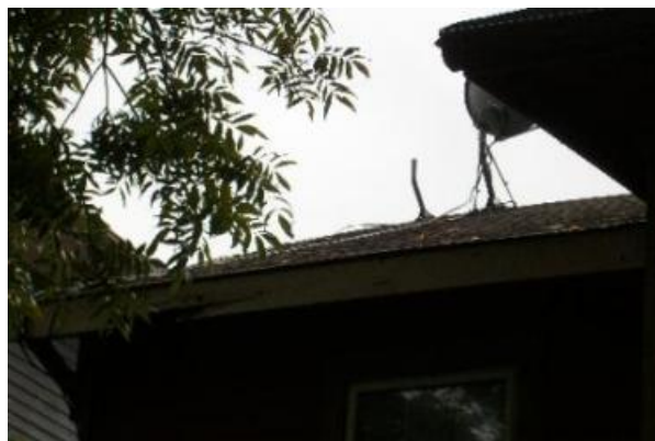
The cables from the Dish are laying on the shingles across the roof
